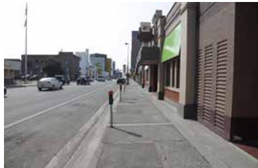
Suspended slab (concrete filled) - 5th Avenue
