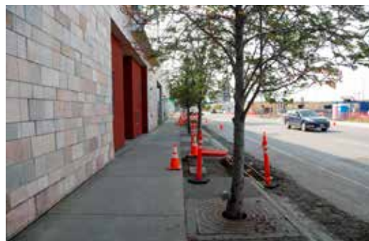
Suspended slab - 4th Avenue at Fire Station
