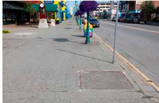
Tree pit (concrete filled) - 4th Avenue
